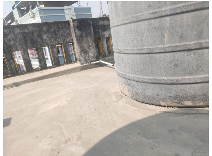
The freshly cemented corner of the roof
