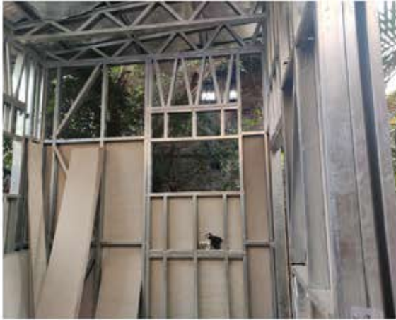
Steel and concrete board structure
